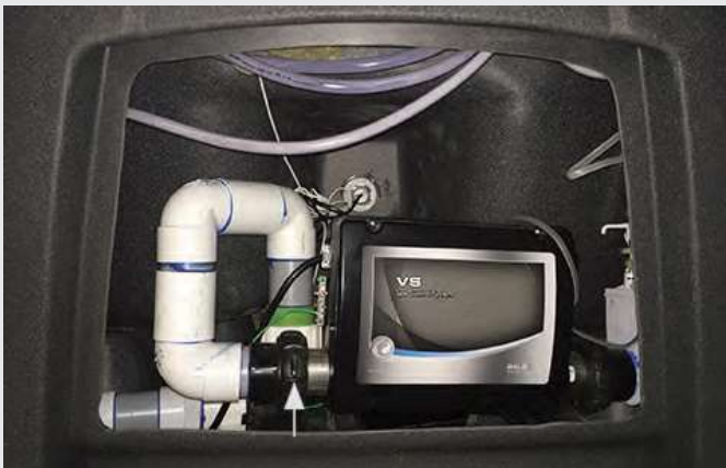
FIGURE 1.9a : HEATER UNION; LOOSEN UP TO BLEED AIR
