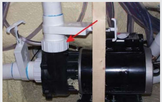
FIGURE 1.9b : PUMP UNION; LOOSEN UP TO BLEED AIR
